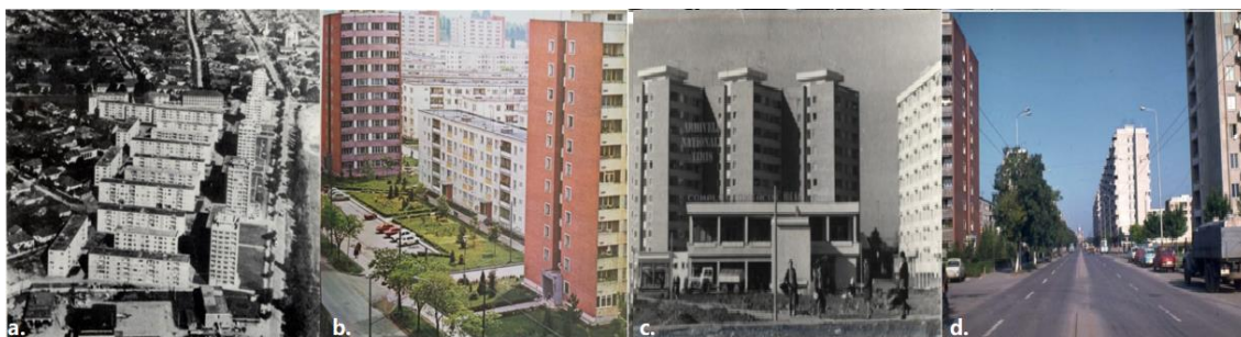
Figure 3. Circumvalațiunii I Area in the early 1970s. a Aerial photo, 1969; b and d. Bd. Gheorghe Lazăr, 1970, 1975; c Favorit Complex in 1974 (source: forumratt.ro)
