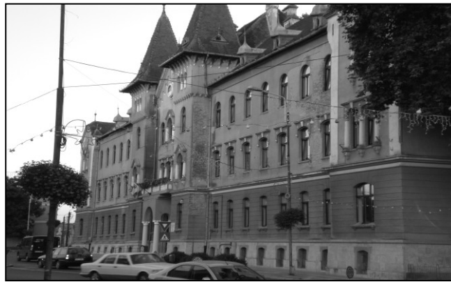
Figure 7: The City Hall from Lugoj in 2008 (foto: Jucu, 2008)
