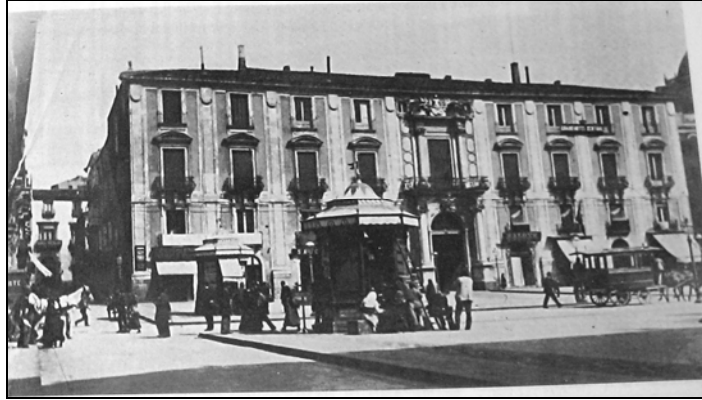
Photo 3: The Palace in 1894 (source: Giarrizzo, 1985, p. 14)
